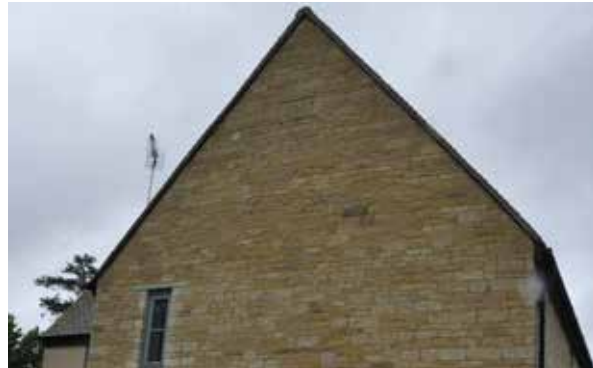
Steeply pitched roof with no overhang, Bletchington
