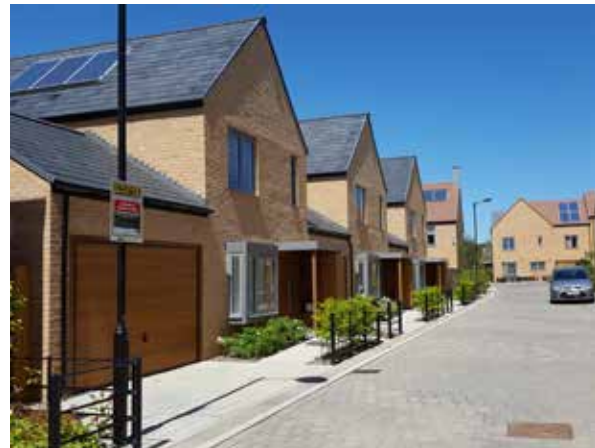
Photovoltaic panels, Trumpington Meadows, Cambridge
