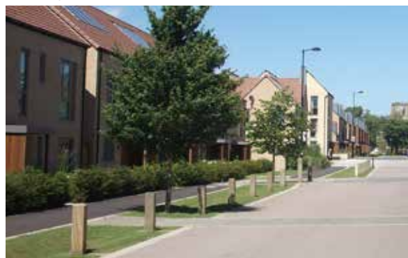
Incorporating SuDS along kerbside, Trumpington Meadows, Cambridge
