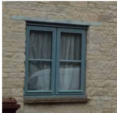
Casement window flush with wall, Bletchingdon
