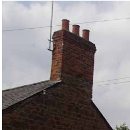
Rectangular brick chimney at edge of ridgeline and central to gable, Bloxham
