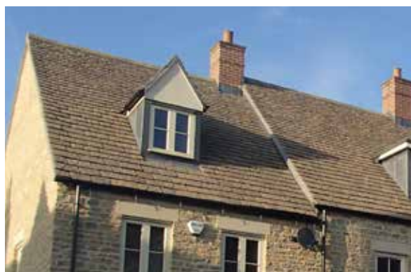
Good examples of modern dormer windows, pitched roofs, slate tiles and brick chimneys, Woodstock
