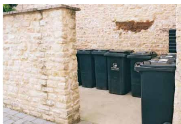
Example of an attractively designed bin store (source: West Oxfordshire Design Guide)
